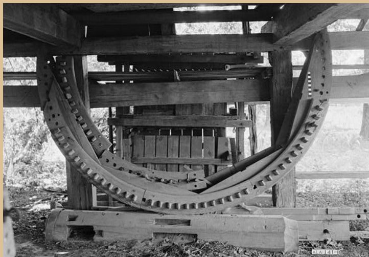
Shaft (on ground) and pinion wheel (in two sections); old gin in background
